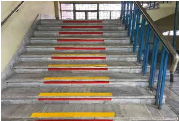
Durable railing along with staircase
