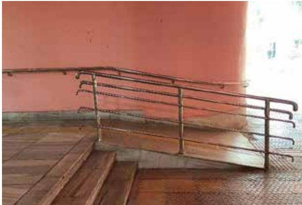
Accessible approach and ramp at building entrance
